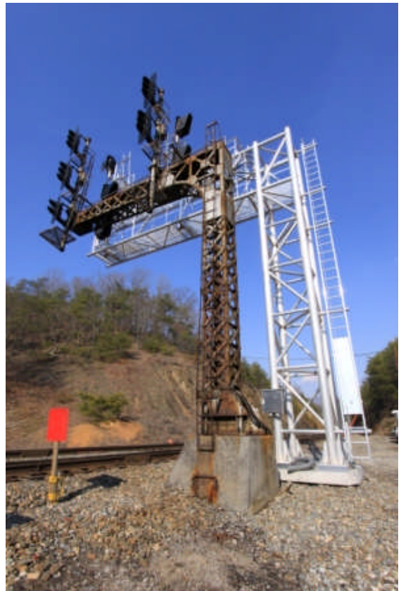
Westbound cantilever with replacement at Chestnut St. 3/12/11
