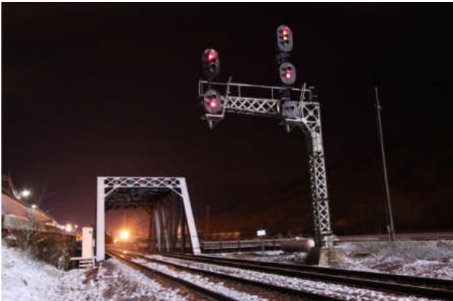
Eastbound cantilever at Jackson River. 12/5/10
