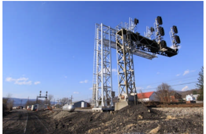
Westbound cantilever with replacement at Chestnut St. 3/12/11
