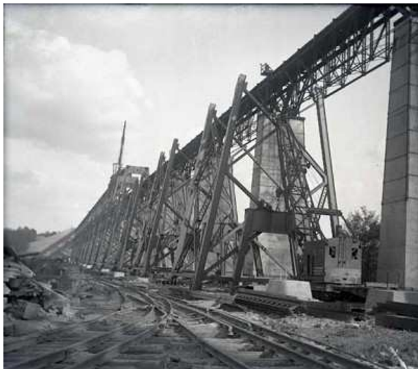
High Bridge construction. c. 1914
